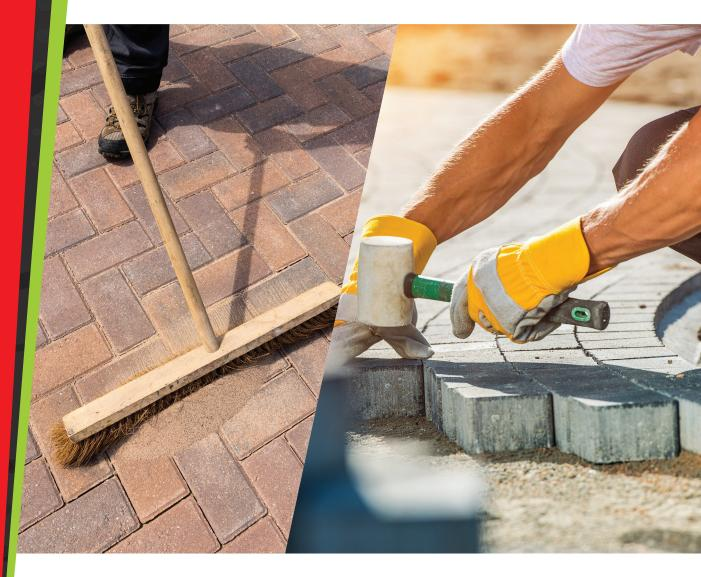
Pavior Sand (also known as Kiln Dry Sand or Jointing Sand) is used for brushing in-between joints of all types of block paving, creating a close and tight bond, adding stability to the block paving.
